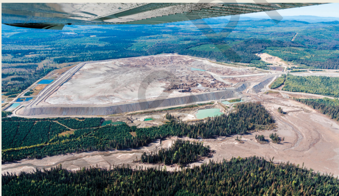
FIGURE 12.1.11 The Mount Polley tailings dam breach caused much destruction in the local environment.
